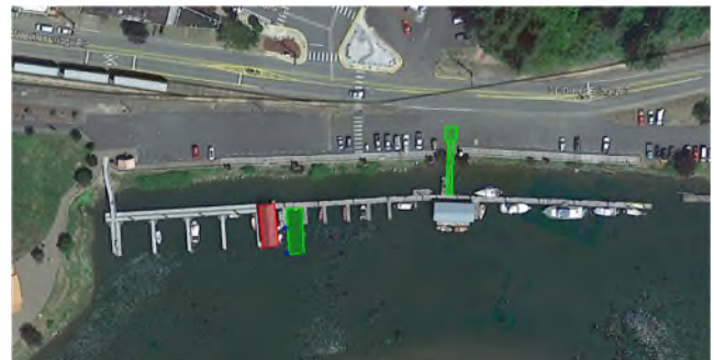
Source: PBS Engineering and Environmental, Inc.
