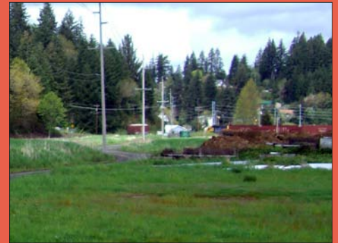
Boatyard is mostly constructed of dredge spoils and modifications will be needed to hold the weight of larger boats and equipment.
