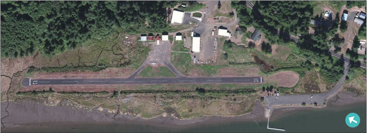
IMAGE 22: Toledo State Airport shown with the Port's Boat Launch & Day Use Area Source: Bing Maps.
