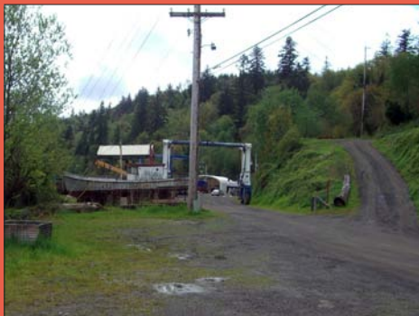
Long, narrow site configuration makes moving and staging larger boats more difficult.
