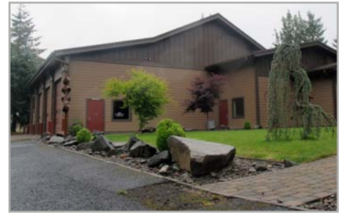
IMAGE 20: Station 1 Office and Lease Space Public art and landscape features added by the Port illustrate a commitment to community aesthetics.
